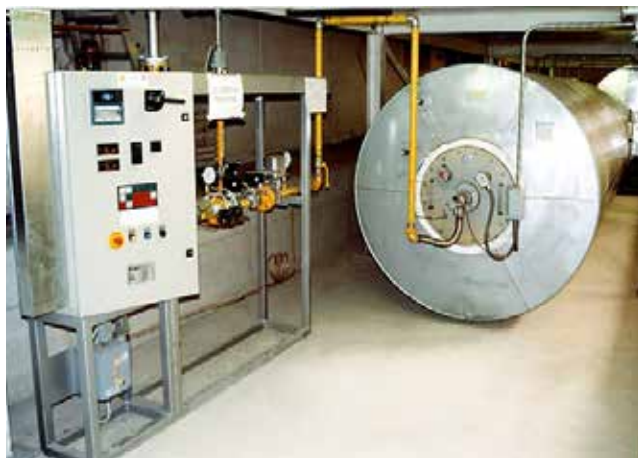
Incinerator (reduction of pollutants in the process air)
