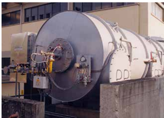
Thermal recuperative post-burner (reduction of pollutants in the process air)
